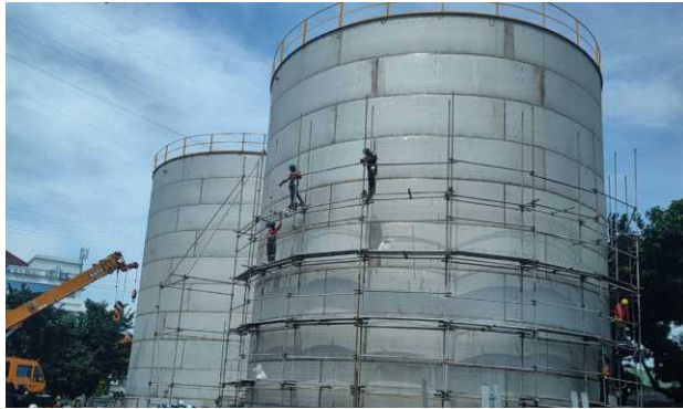
Project Epc Filling Plant PT Industri Nabati Lestari
