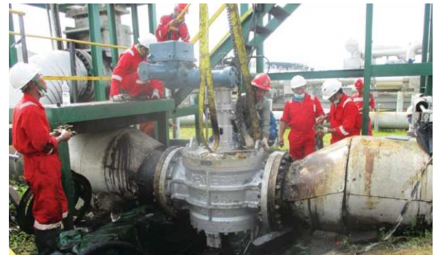
Repair Valve Pertamina EP
