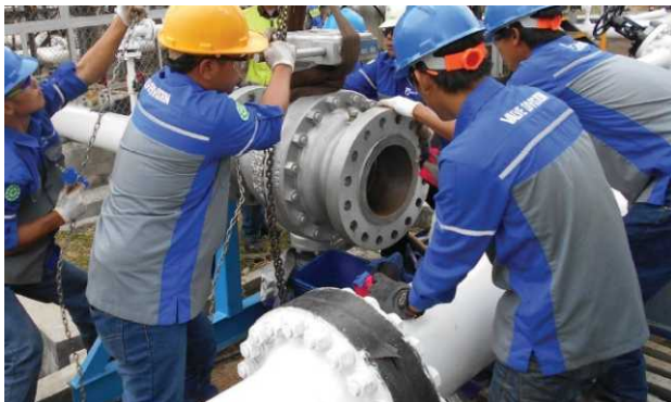
Repair Valve TBBM Padalarang
